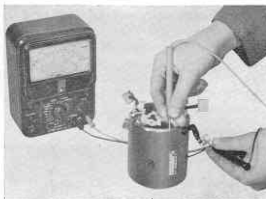
Fig. EE-61 Testing for Ground
